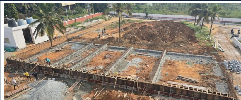
Courtyard — footings cast, plinth beams and lift pit in progress
