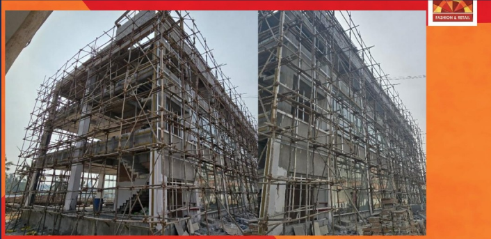
Façade — three-side glazing on Block A behind full scaffolding
